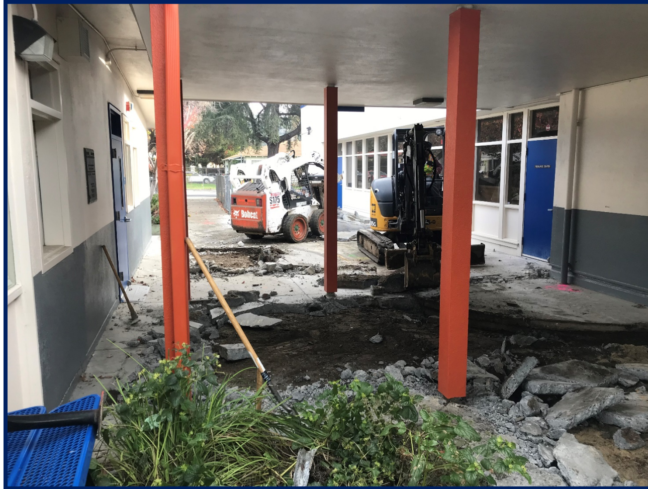
Toyon – Site Work Before
