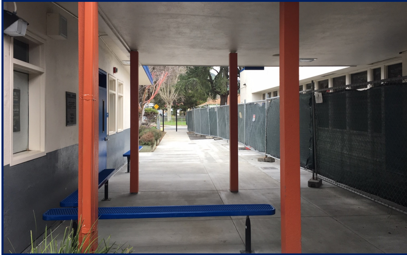
Toyon – Site Work After
